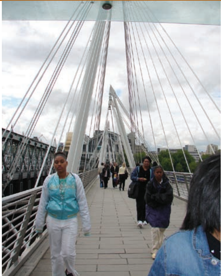
The Hungerford Bridge features both pedestrian and rail access between Charing Cross Station and the South Bank Centre.
