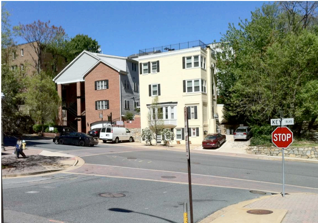
Figure 9: Traditional Multi-Family Housing along Key Boulevard at North Nash Street
