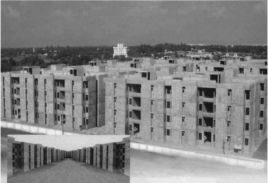
Figure 7.5 Low-Income Housing Built by AUDA on Land from the Prahlad Nagar TPS
