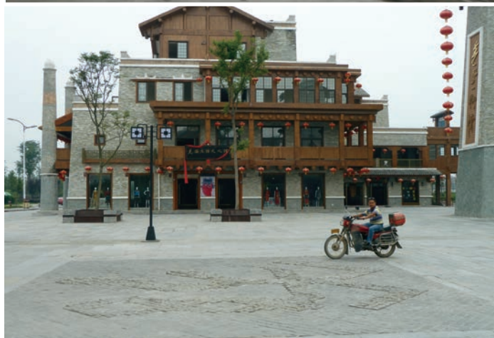
Buildings toppled and rebuilt following the 2008 Wenchuan earthquake in China.
