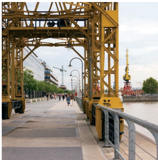
Harbor cranes are still an integral part of the cityscape.
