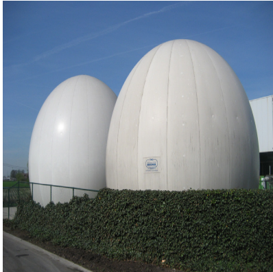
Figure 6: Anaerobic Digesters (Arup)
