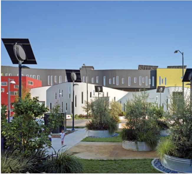
Tassafaronga Village in East Oakland, California, set a new standard for energy-efficient, beautifully designed affordable housing when it opened in 2010. Credit: David Baker Architects.
