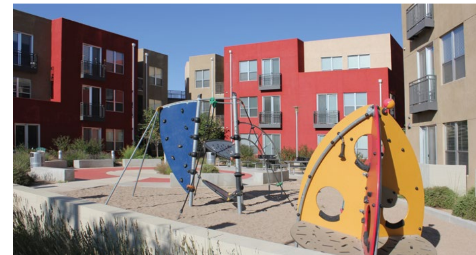
Above: Dudley Neighbors CLT in Boston provides affordable housing and community control of land on behalf of its founding organization, the Dudley Street Neighborhood Initiative (DSNI), freeing DSNI to focus on community planning and organizing. Credit: Travis Watson
