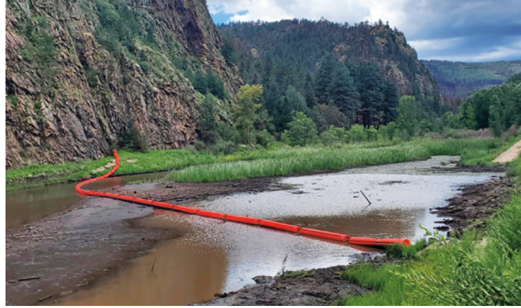
Flood control in the areas affected by the Hermits Peak–Calf Canyon fire included the installation of temporary dams (left) and floating barriers to slow or stop large pieces of debris (right). Credits (left to right): U.S. Army Corps of Engineers, U.S. Forest Service.
