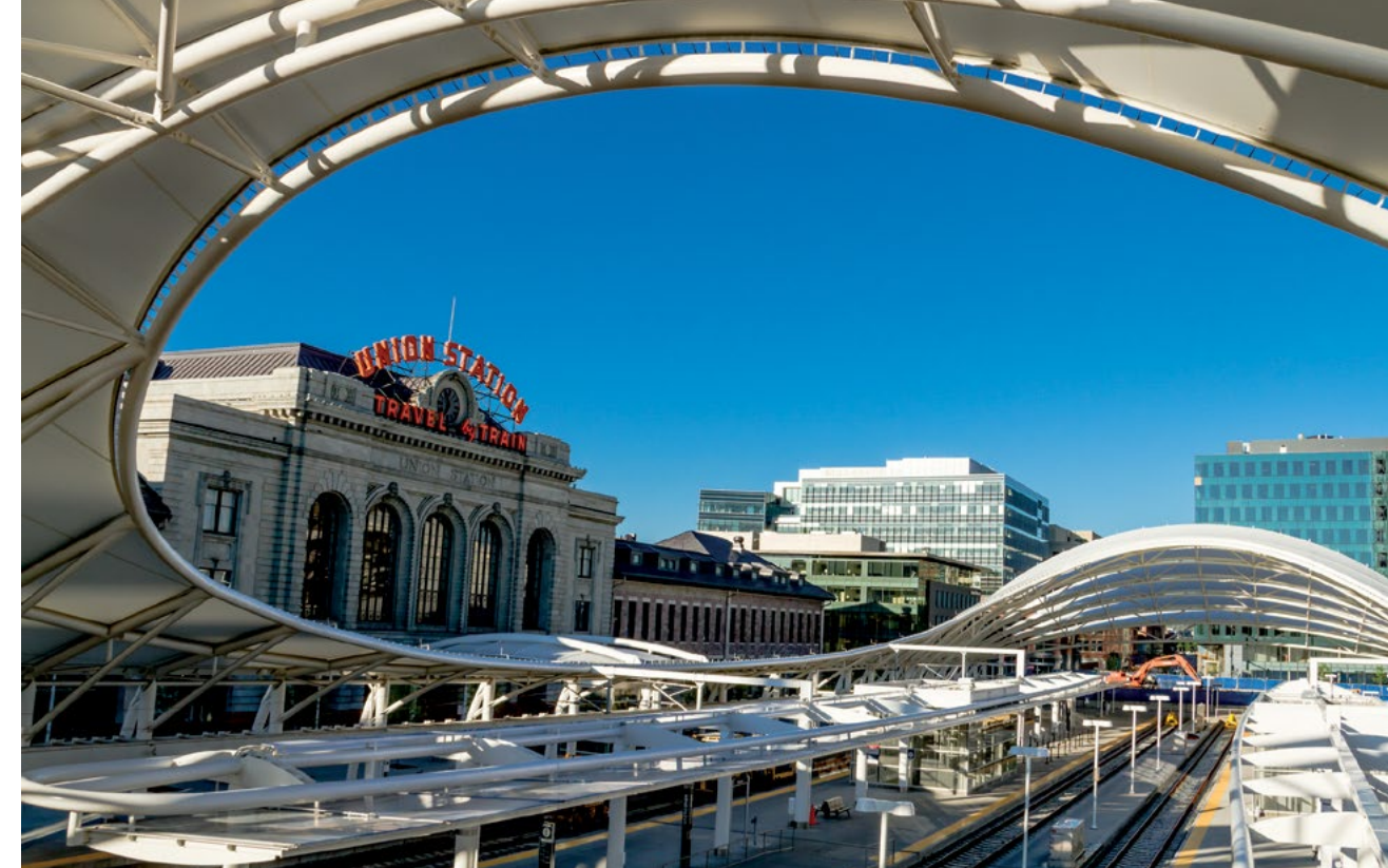
Denver’s newly restored Union Station has attracted $2 billion infrastructure and mixed-use development. Credit: tvirbickis/iStock
