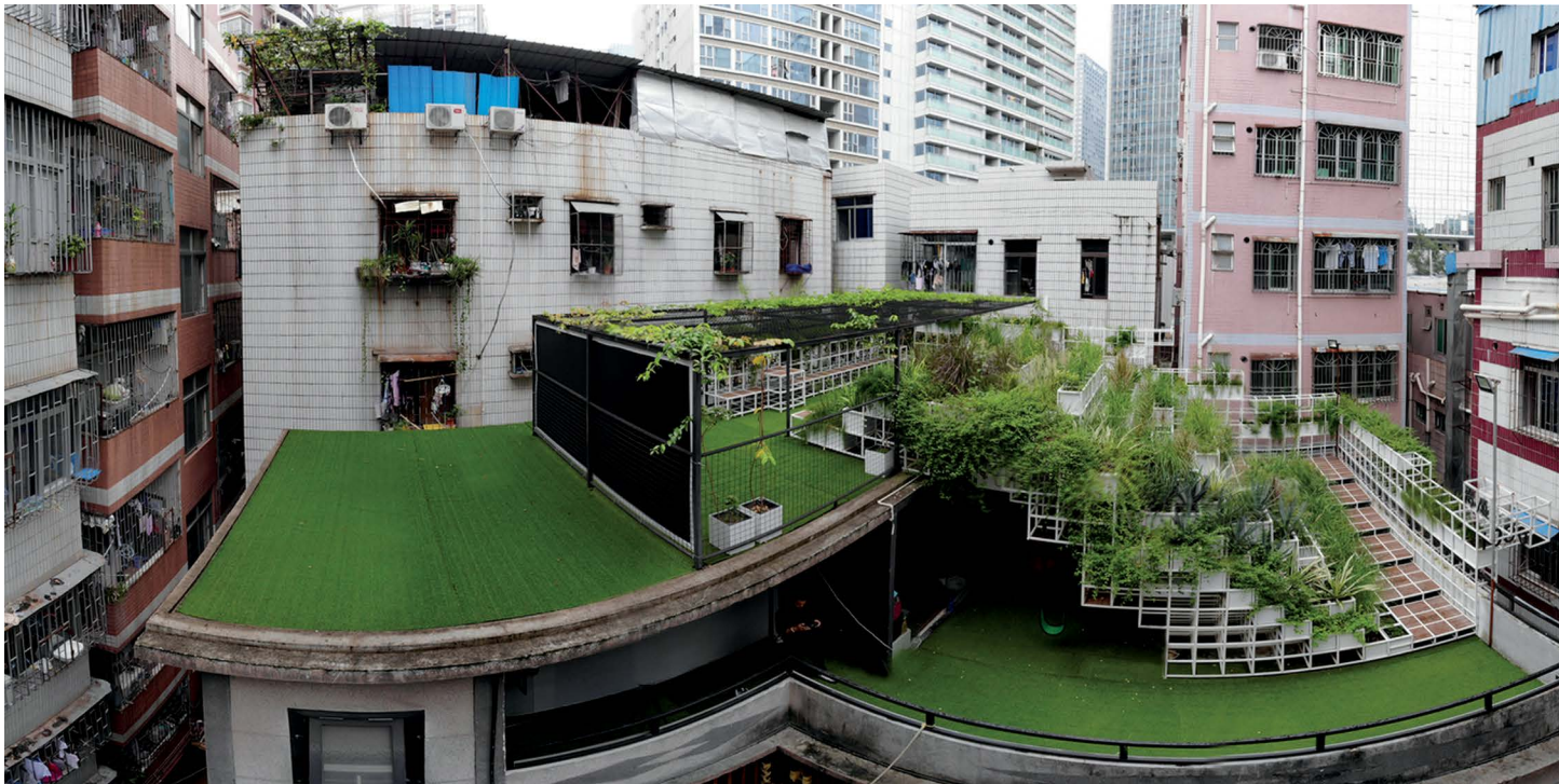
The Nature Conservancy's green roof project in the urban village of Gangxia catches over 65 percent of the rain that falls on it. Credit: John Siu.
