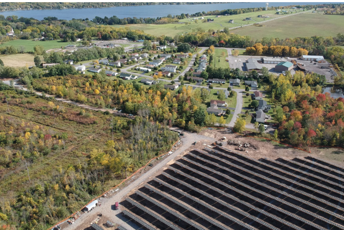
Homeowners in Lakeville Village, a resident-owned community in Geneseo, New York, opted to install a solar array on 20 acres of their land, which they leased to a renewable energy company. Credit: ROC USA.
