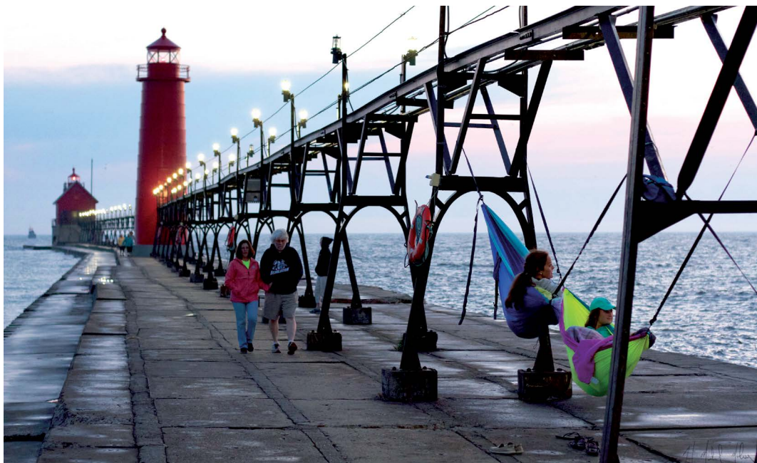
The Grand Haven waterfront is a draw for tourists and residents alike. The city's new master plan includes regulatory and infrastructure policies aimed at protecting it from the worst impacts of climate change. Credit: H. Michael Miley via Flickr CC BY 2.0.
