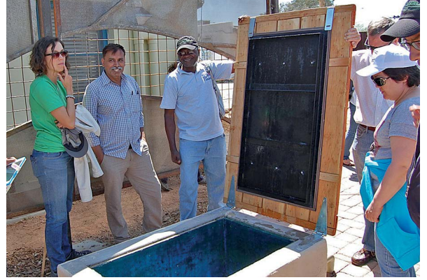
Visitors to the Watershed Management Group's Living Lab and Learning Center in Tucson peer into the 10,000-gallon underground cistern the organization uses to capture and store rainwater. Credit: Watershed Management Group, watershedmg.org.
