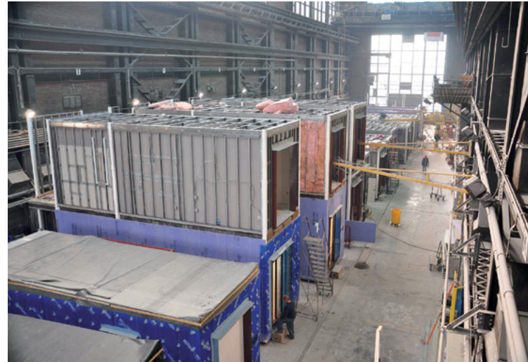
Carmel Place, New York's first micro-unit apartment building, features modular units that were built in a factory space at the Brooklyn Navy Yard (left), then pieced together on-site on a lot considered too small for traditional construction (right). Credit: nArchitects.
