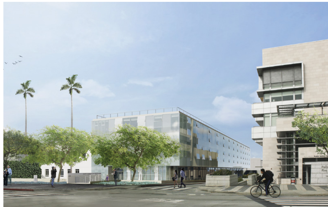
Santa Monica's new City Services Building will consolidate municipal operations while aspiring to be one of the greenest buildings in the world. Credit: Frederick Fisher and Partners
