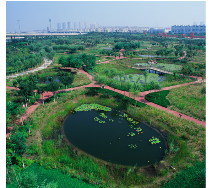
On the site of a former garbage dump in Tianjin City, China, Turenscape's Tianjin Qiaoyuan Wetland Park features paved pedestrian paths and a rainwater pond designed to irrigate vegetation that remediates saline-alkali soil. Photograph by Kongjian Yu.
