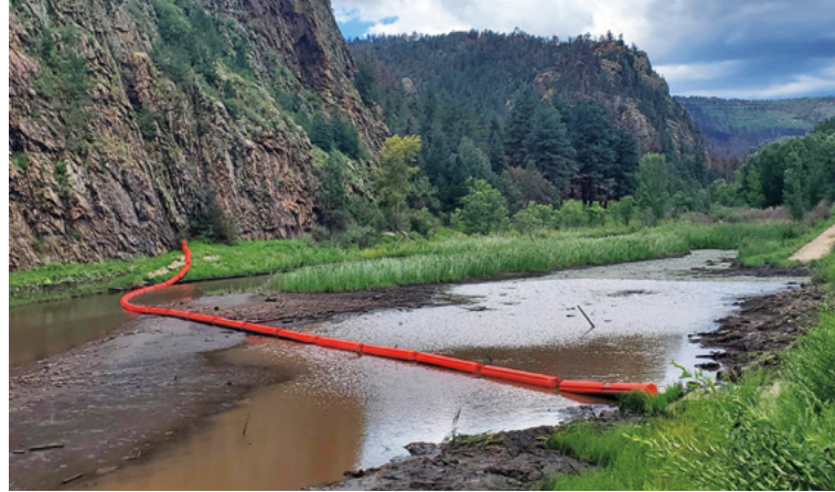
Flood control in the areas affected by the Hermits Peak–Calf Canyon fire included the installation of temporary dams (left) and floating barriers to slow or stop large pieces of debris (right). Credits (left to right): U.S. Army Corps of Engineers, U.S. Forest Service.
